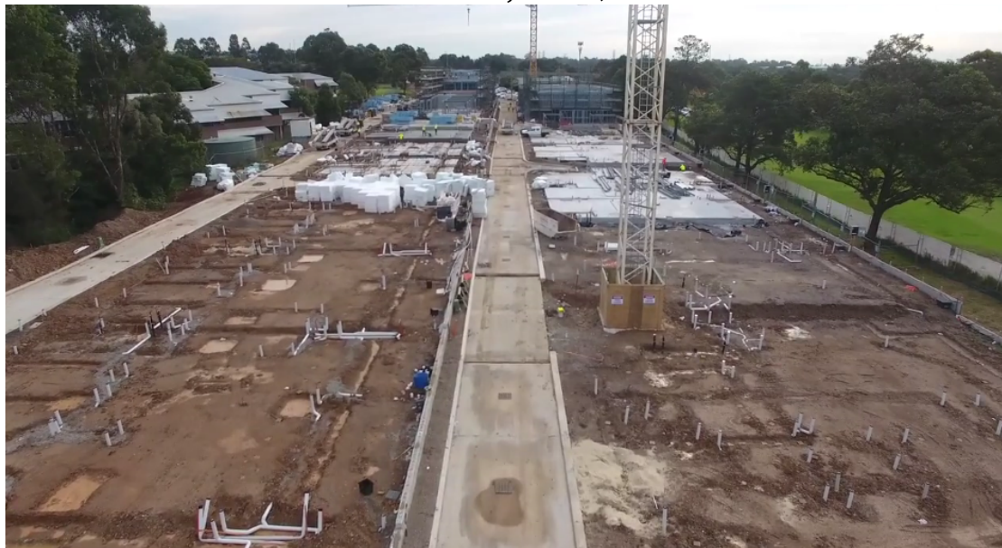
Metro townhouses under construction – June 16, 2017
